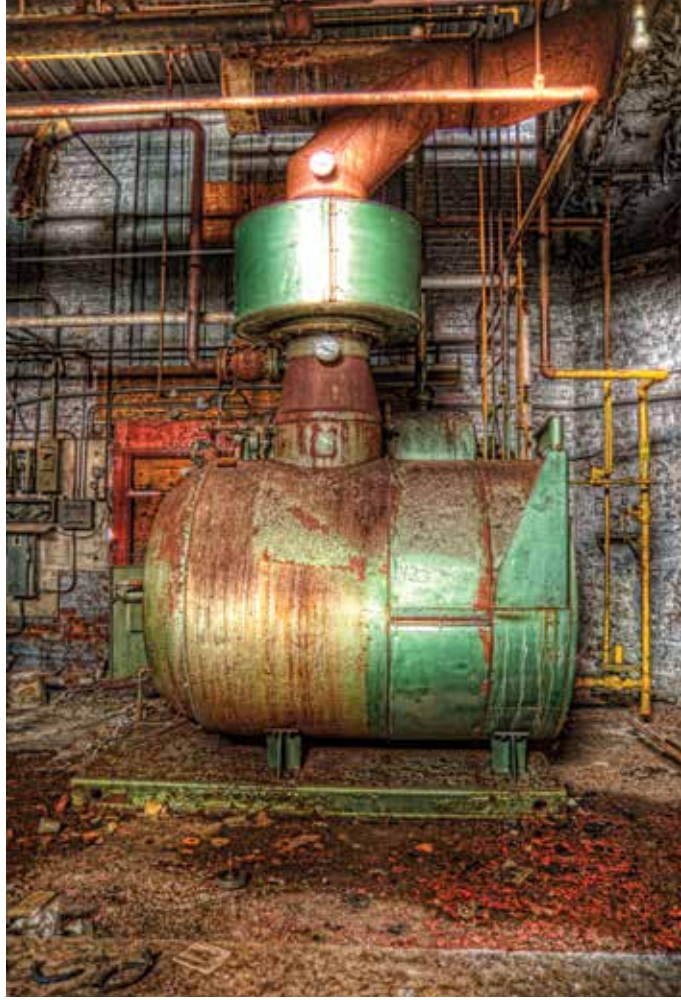
▲ “RUSTING AWAY” This was also taken at the Harvey Woods Factory. This old furnace was in the basement, and I loved the colours in the rust. I enhanced the vibrancy to help strengthen the rust effect in the photo and used some filters to help in the process.
